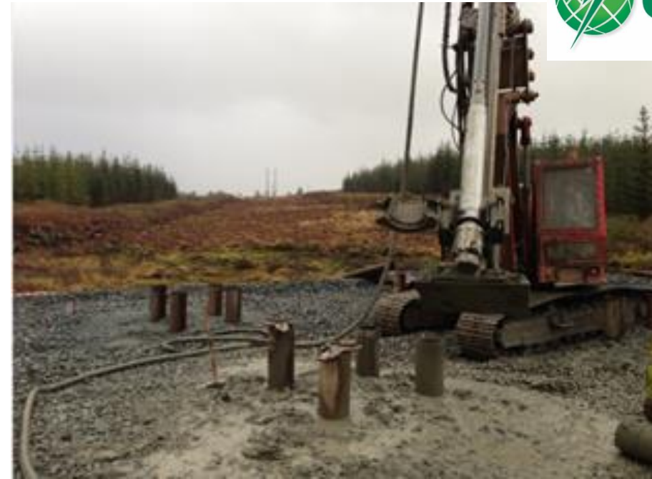
Pile installation
