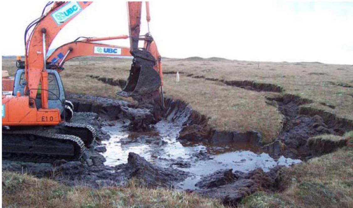
Excavation in Peat
