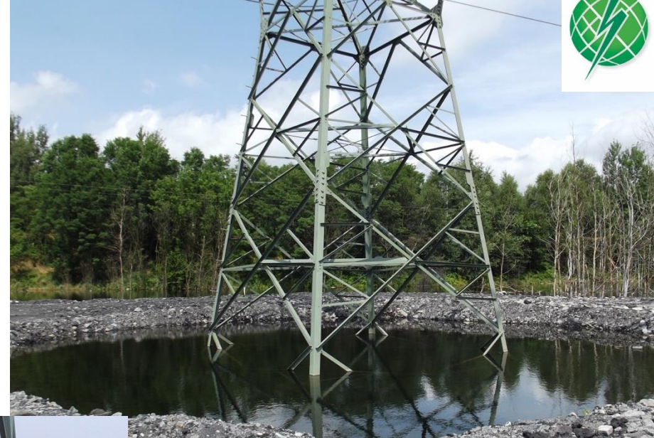
Tower 220kV plunged in water 5 m deep
