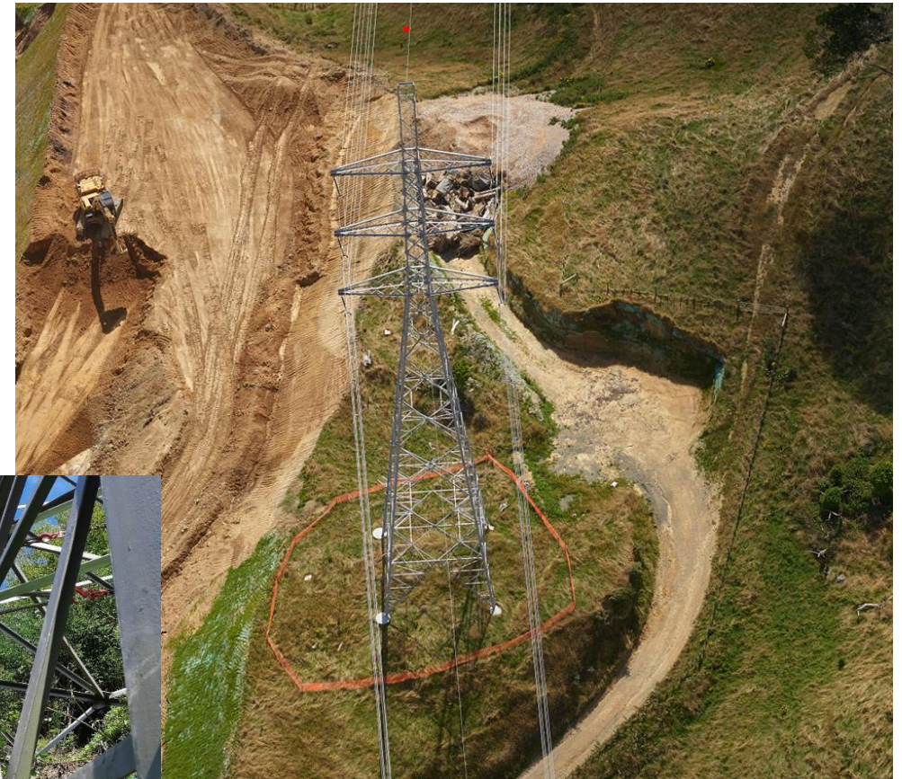
Cut excavation near the tower (New Zealand)
