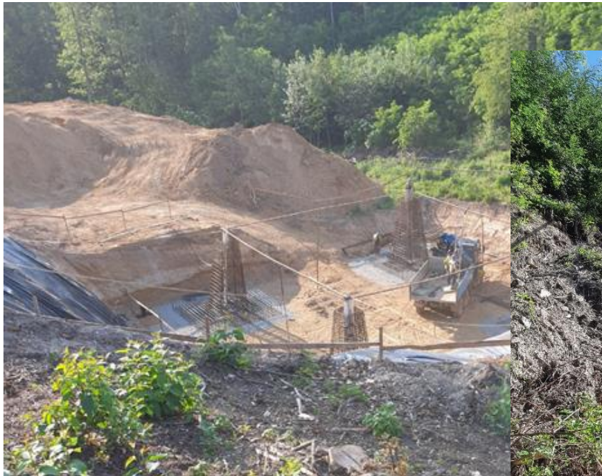
Execution of the foundation on the slope (Poland)
