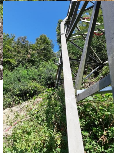
Damage of the tower structure (Slovenia)
