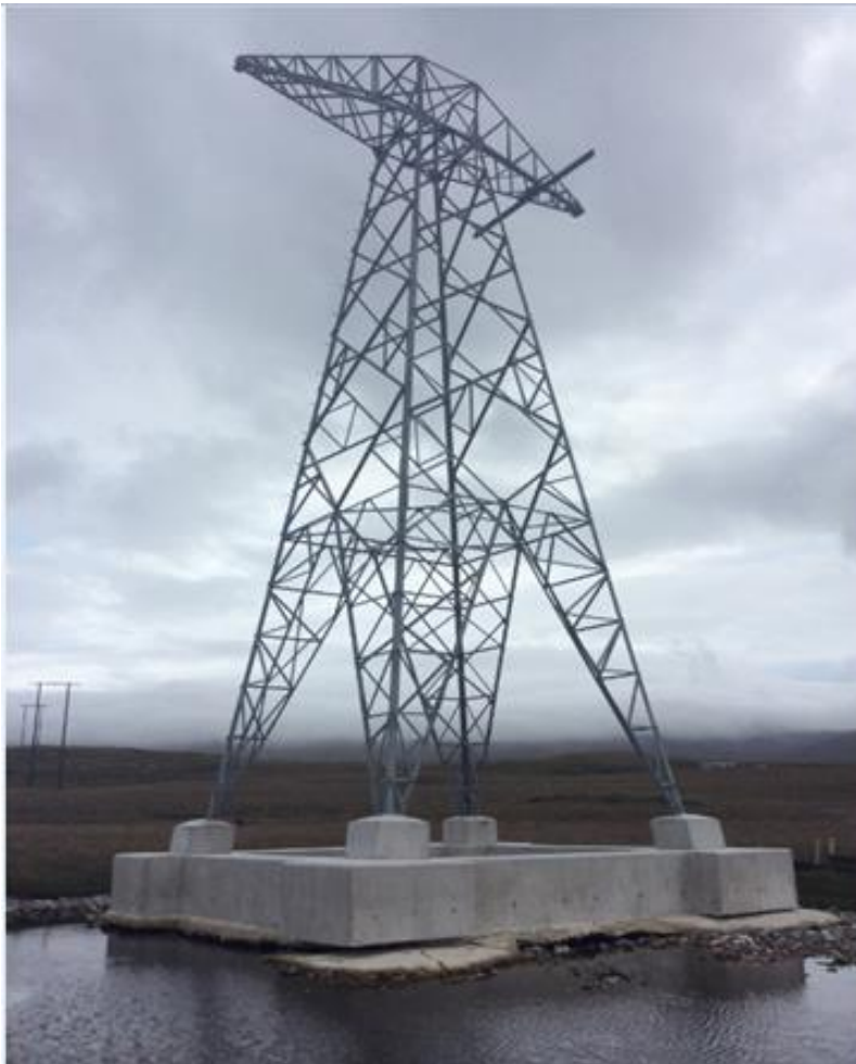
110kV Tower (Ireland)
