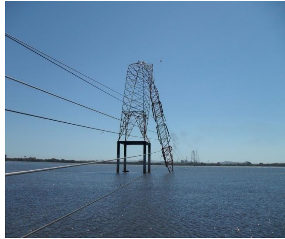
Line 2x220 kV, piles deep foundations (Chile)
