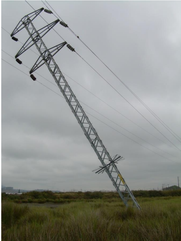
Line 2x66 kV, monobloc foundation (Chile)
