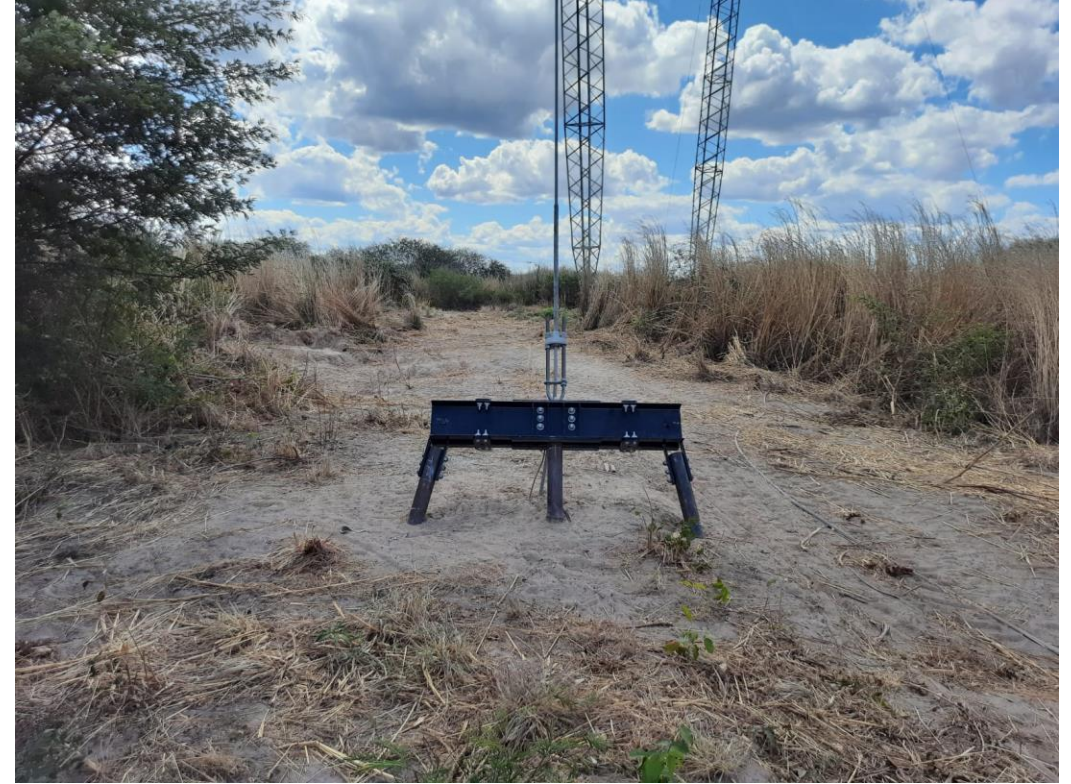
Installation of the helical piles to connection on the structural beam (Brasil)
