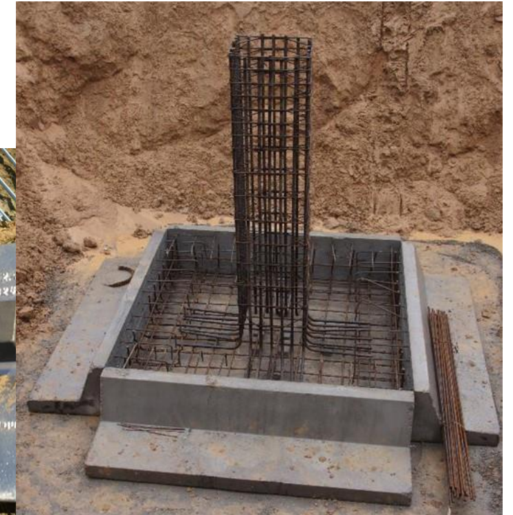
Innovative precast-monolithic foundations (Poland)
