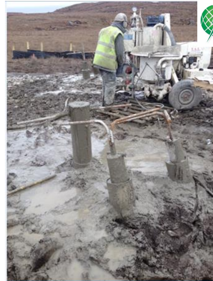
Piles installed showing outer sacrificial casing and inner CHS (Ireland)
