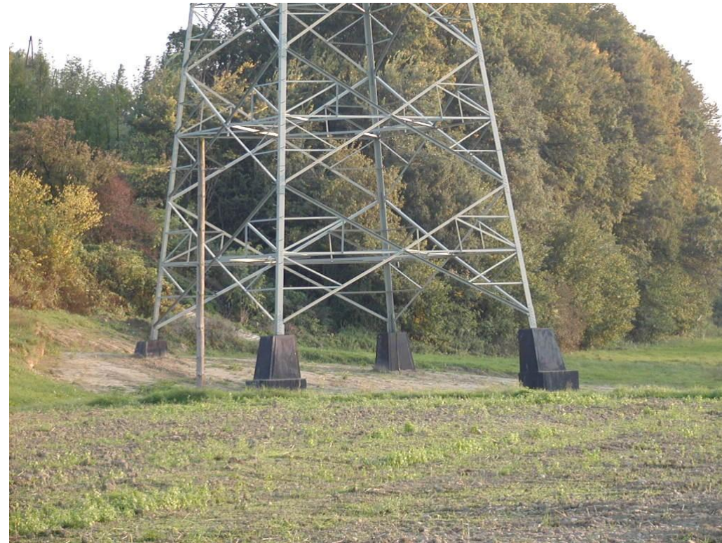
Tension tower, pile foundation (Franki piles),
